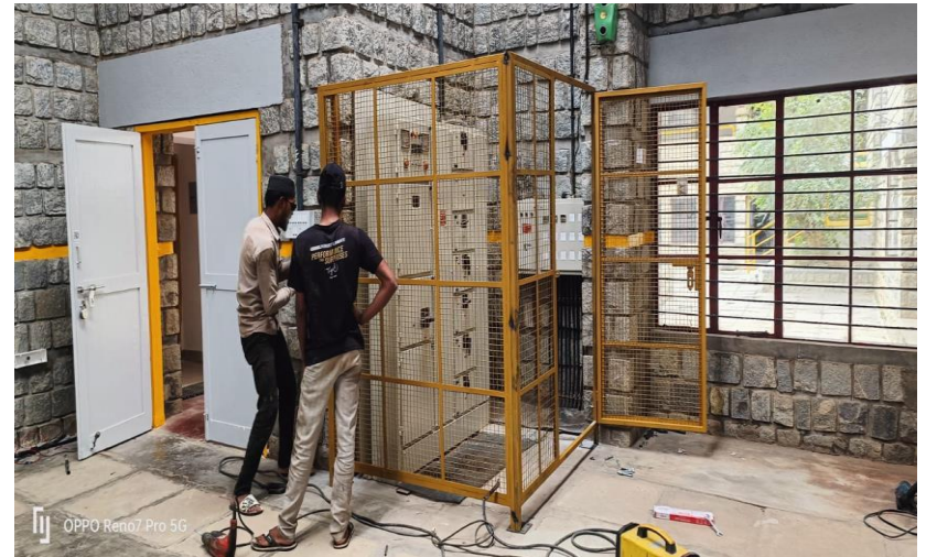
Electrical Work at warehouse
