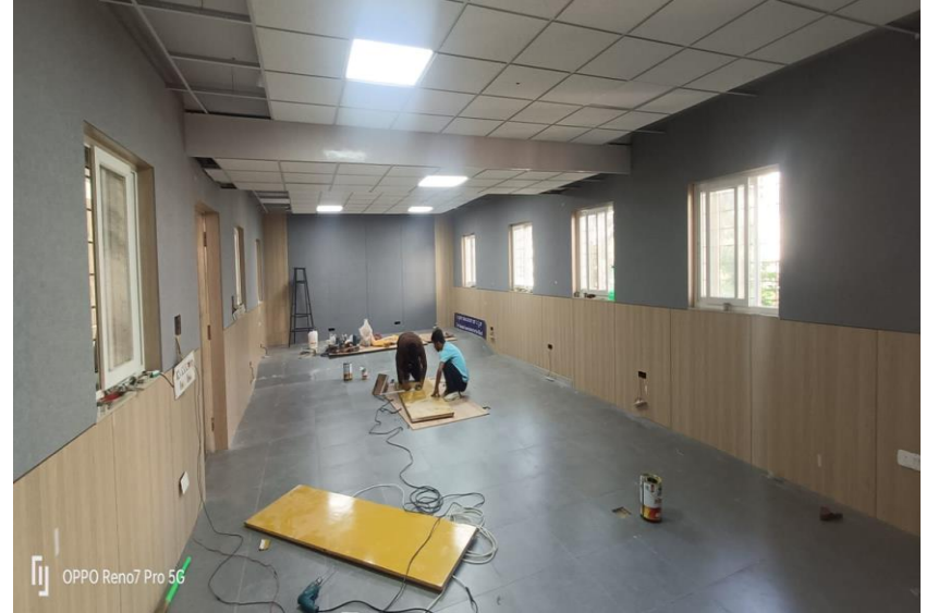
Renovation of conference Room
