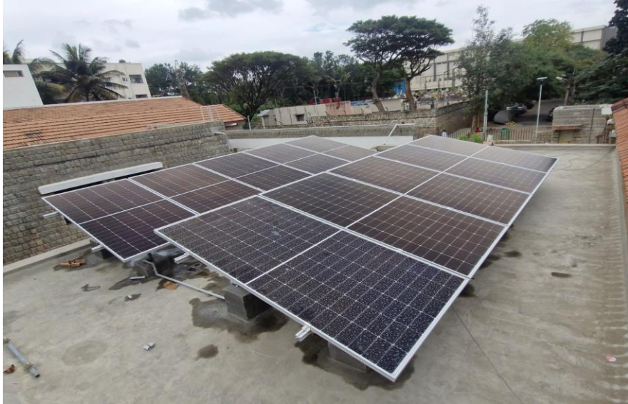
Solar panel installed at NABK
