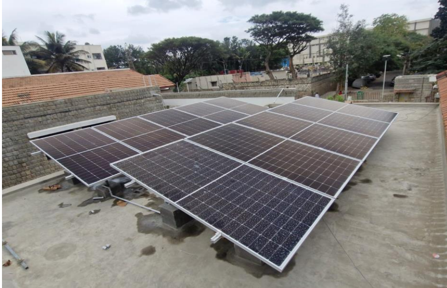
Solar panel installed at NABK
