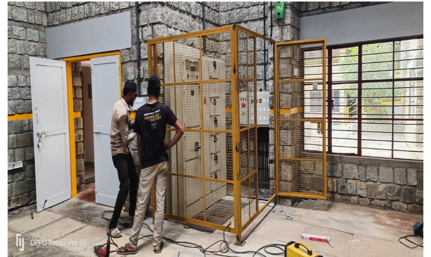
Electrical Work at warehouse
