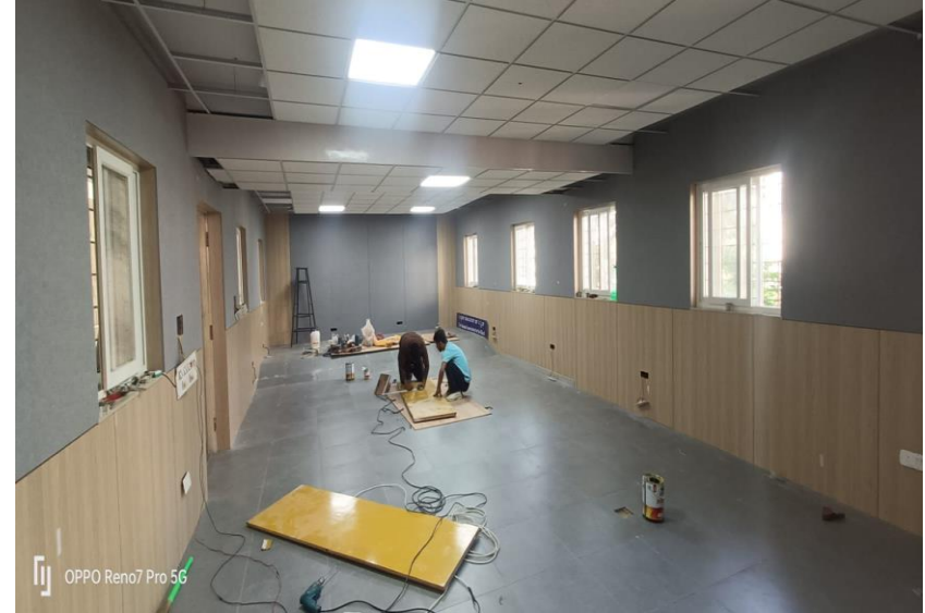
Renovation of conference Room
